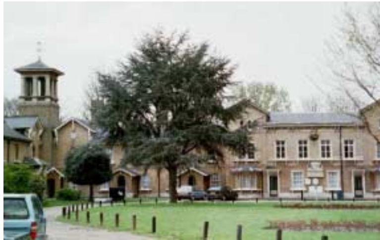
Figure 1. The Almshouses situated on the Lea Bridge Road
