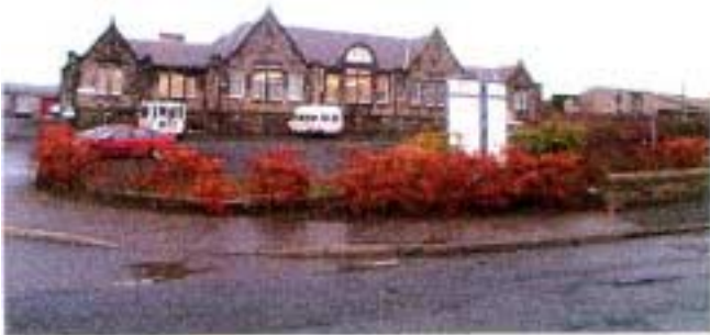
A front view of the building
